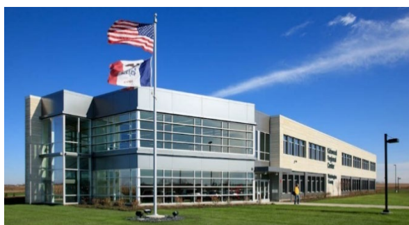
Kirkwood Washington County – Design Engineers, Bid 3/13
